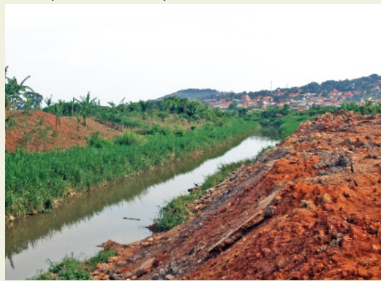
Photo 9: Land filling in a wetland in preparation for industrial construction in Kampala City
